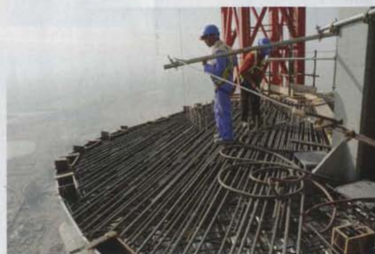
The tower used over 430,000 cubic yards of concrete and 43,000 tons of steel rebar. To help determine the concrete-to-rebar ratio, three-dimensional finite-element analysis models were used to predict the effects of creep and shrinkage.
